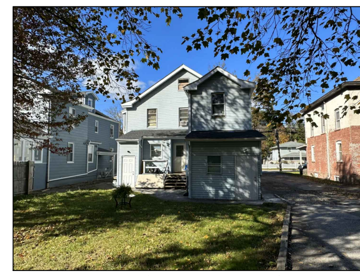
EAST FACADE (REAR OF BUILDING)
