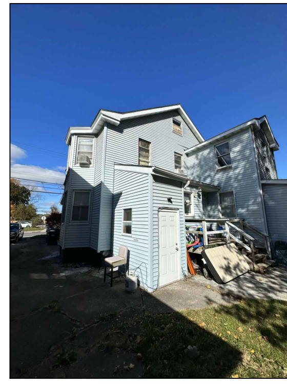
SOUTH EAST CORNER
