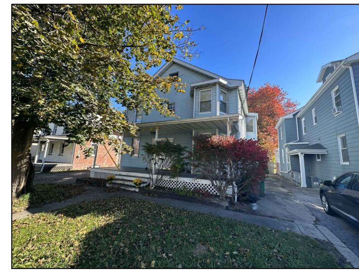
WEST/ FRONT FACING SOUTH AVE
