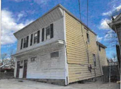
PHOTO OF EXISTING FRONT ELEVATION
